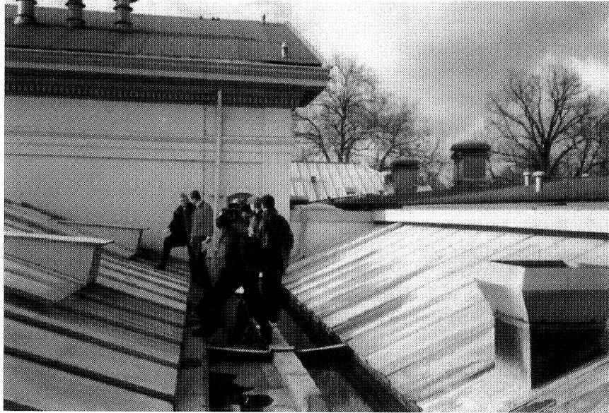
FIGURE 1. Observation of the aquarium roof.
